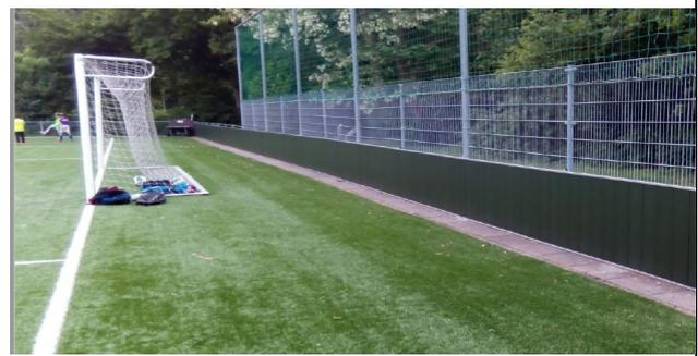
Fence barrier to contain infill within the field area<sup>19</sup>
