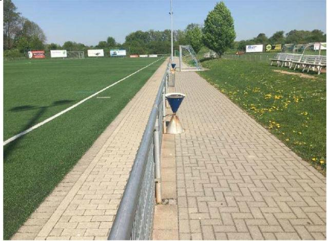
Profiled paved margins to separate synthetic turf from surrounding environment<sup>22</sup>
