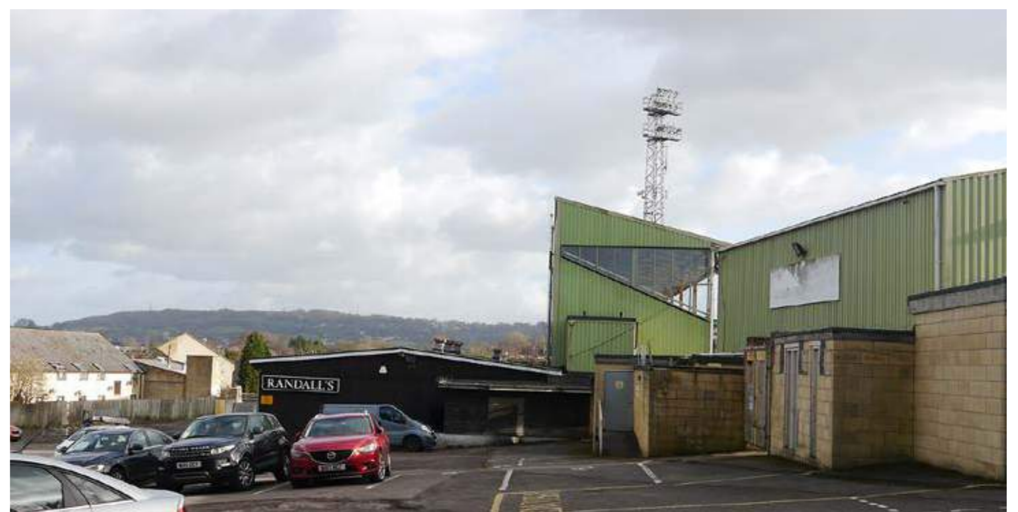
Randall's Bar and main grandstand
